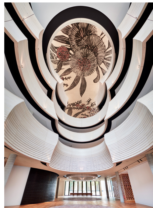
Stepped plywood balustrades in Monash Chancellery
